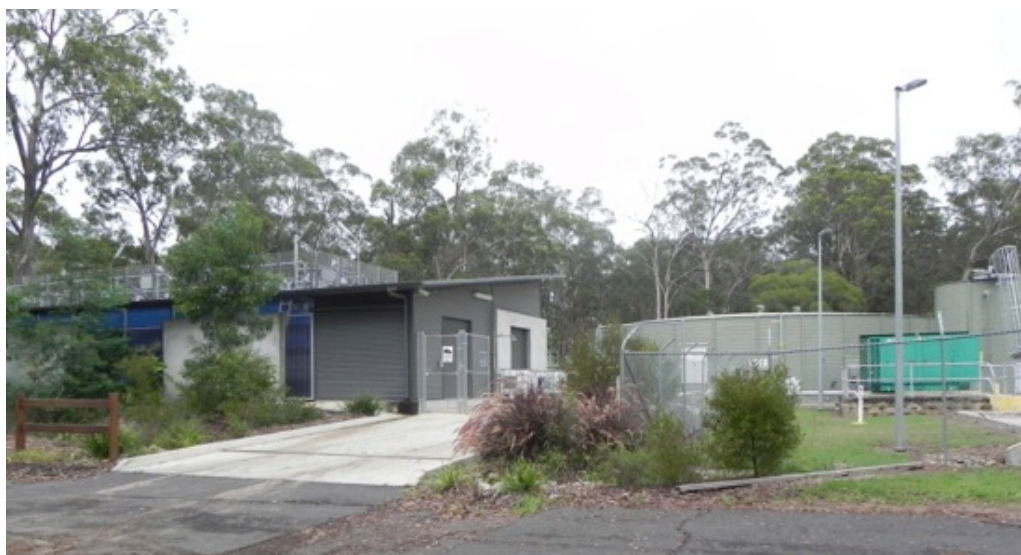
Figure 8 - The water recycling plant at Pitt Town Local Water Centre
