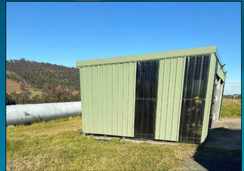
Temporary PAC Dosing Facility Upstream of Dungog WTP
