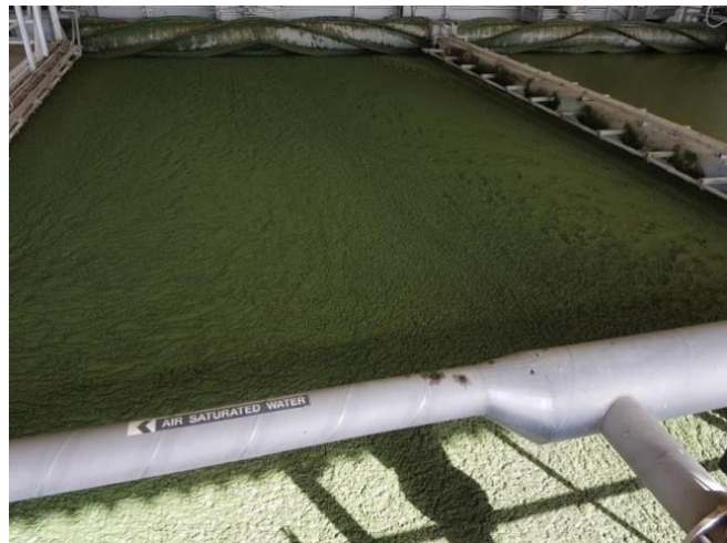
Cyanobacteria accumulation inside DAF sludge
