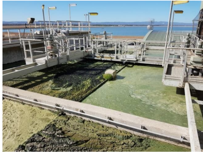
Cyanobacteria breakthrough into flocculation system
