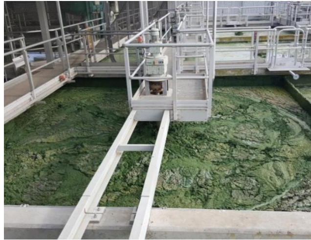
Cyanobacteria breakthrough into mixers
